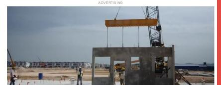
W-PC is a prefabrication method in which large concrete panels are assembled on-site
