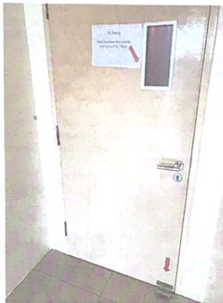
Nestle converted the doors at its HQ to be foot operated.
